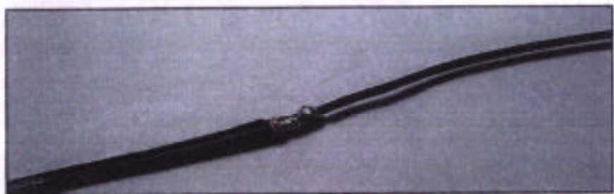
Photo C— Connection of outer end of coax section (farther from center). Note that both center conductor and shield are connected to the wire.
